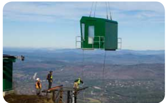
Installation of Mittersill Chairlift
