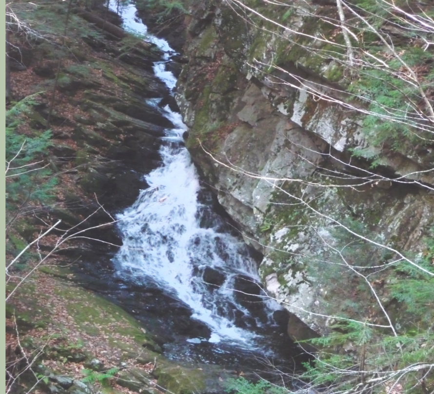
Fig. 2. Sheeting fractures dipping southwest (to the right) in the stream channel.
