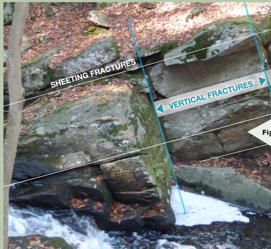
Fig. 3. Two sets of vertical fractures, intersecting the horizontal sheeting fractures.
