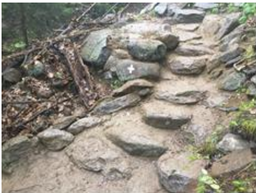
Rock staircase constructed on the White Cross Trail during one of five hitches at Monadnock SP.
