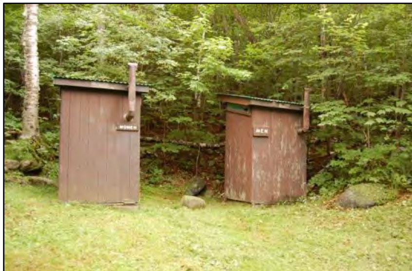
Wiley House Site, Pit Toilets Source: PAL, 2013
