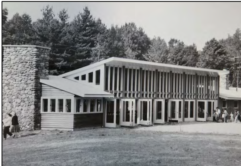
Addition to Mt. Sunapee base building
