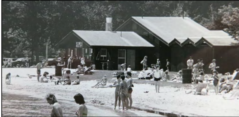
Mount Sunapee State Park (lakeside elevation before alterations)
