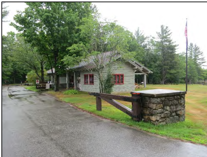
Administration Building, Moose Brook State Park, Gorham (1937-8)
