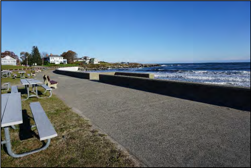
Concrete sidewalk behind concrete seawall, Wallis Sands State Park
