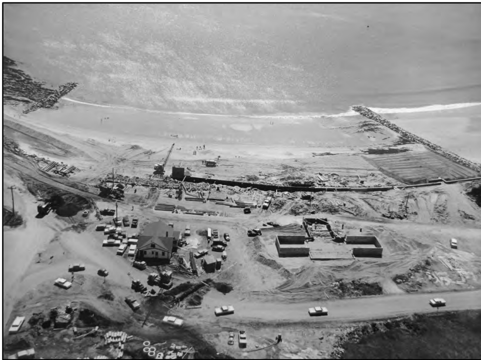
Wallis Sands State Park under construction, 1963
