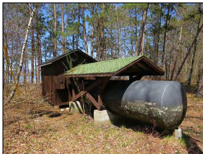
Wellington State Park Pump House, 1949
