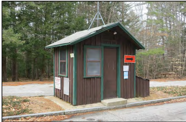
Pawtuckaway State Park Contact Station, 1966
