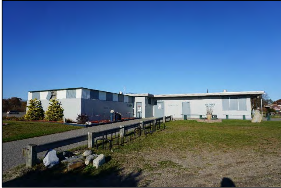
Wallis Sands State Park, Rye, 1964 (bathhouse portion is at left in photo)
