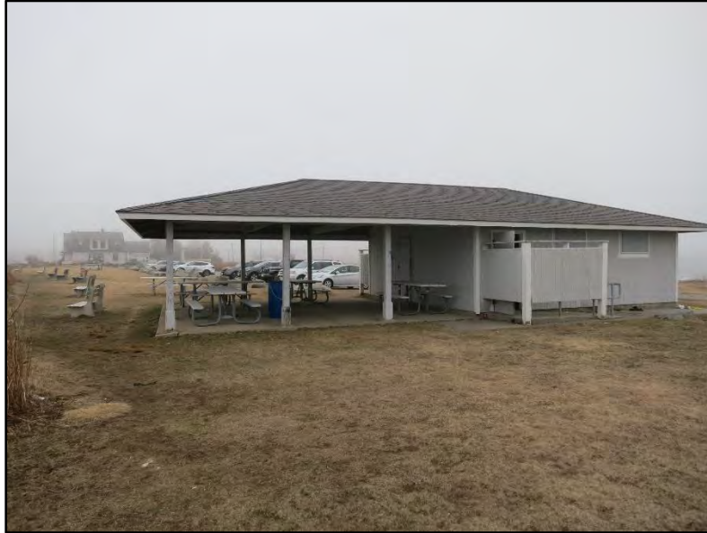
Toilet Building/Picnic Shelter, Ragged Neck Picnic Area, Rye Harbor State Park, 1965
