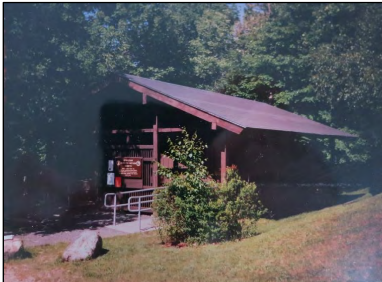
Toilet Building/Shelter, Winslow State Park, 1965
