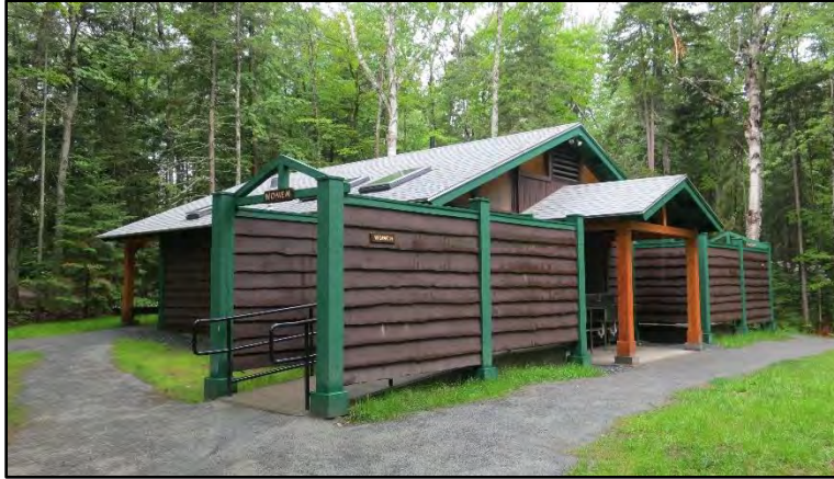
Shower/toilet building, Moose Brook State Park, 1973
