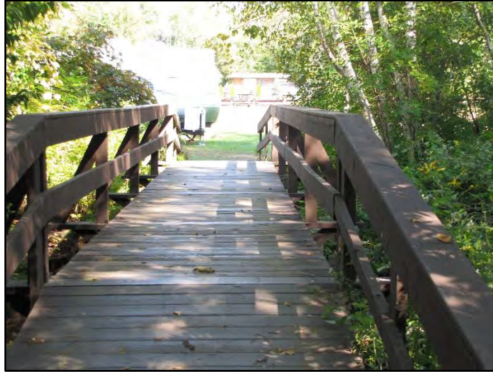
Footbridge over Poor Farm Brook
