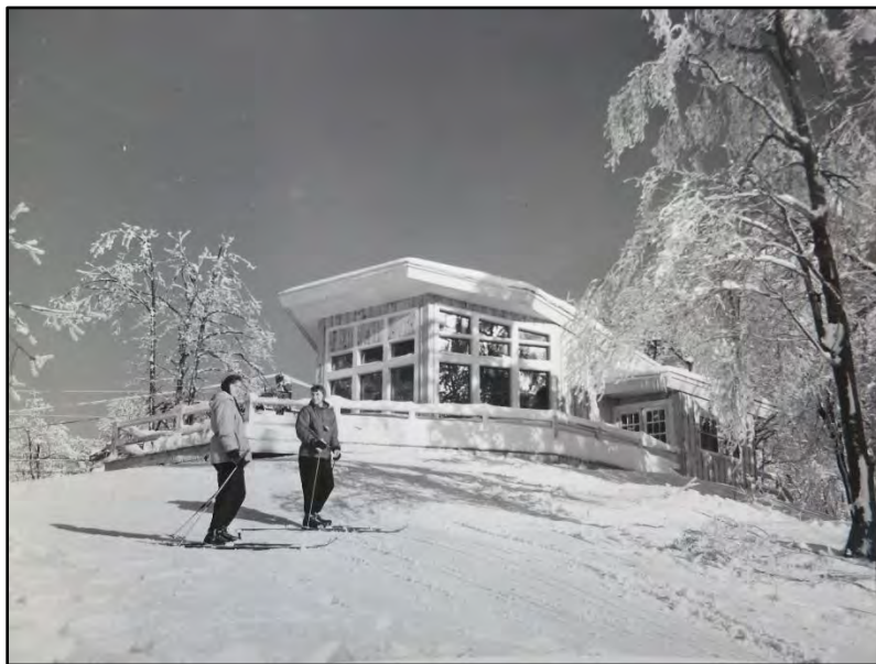
Mountain Shelter, Mt. Sunapee State Park
