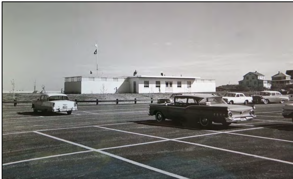
Wallis Sands State Park main building shortly after construction, 1964
