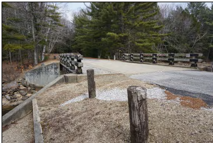
Bridge, Pawtuckaway State Park
