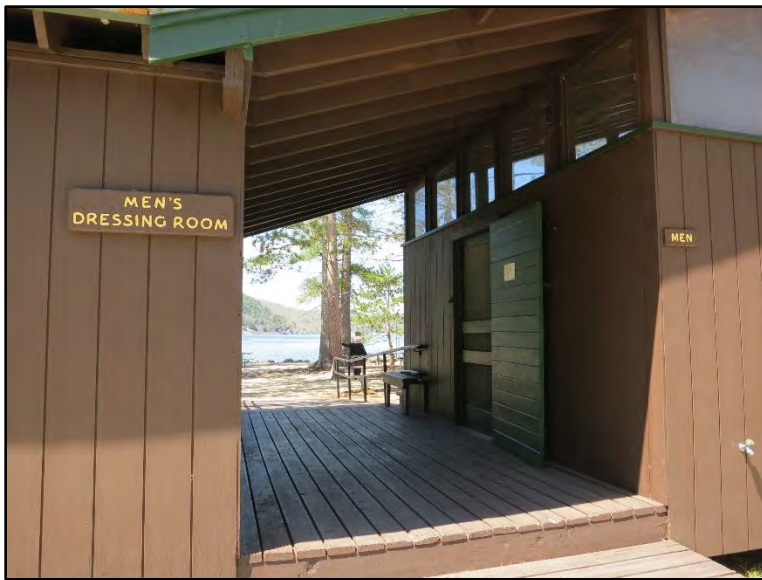
Wellington State Park Bathhouse, 1969
