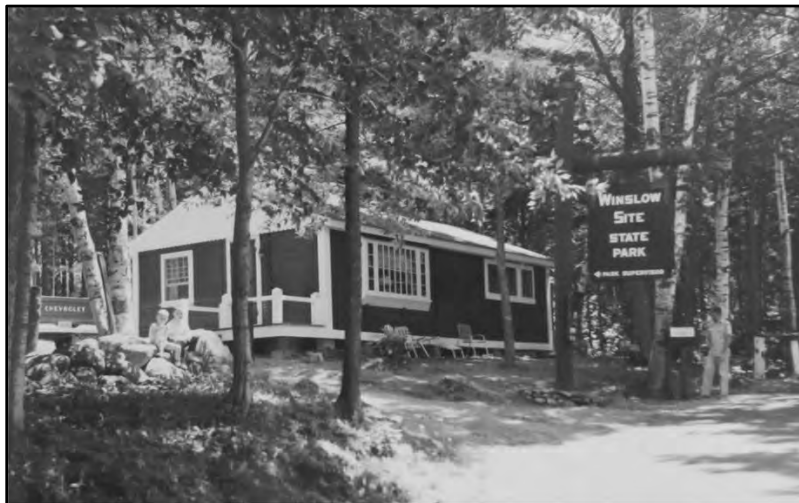
Historic view, Manager's cottage, Winslow State Park
