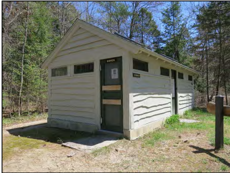
Toilet Building, Wellington State Park, 1962
