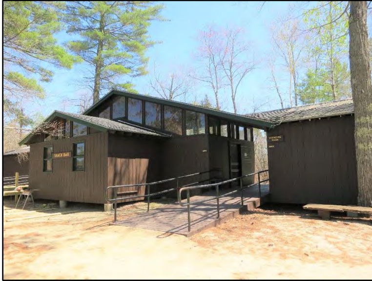
Wellington State Park Bathhouse, 1969
