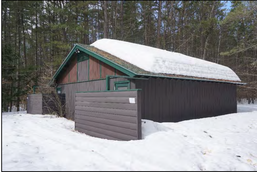
White Lake State Park Shower Building, 1977
