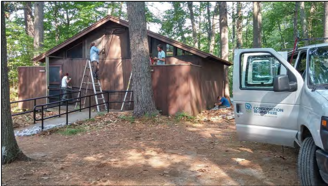
SCA workers at Campers Beach, Greenfield State Park
